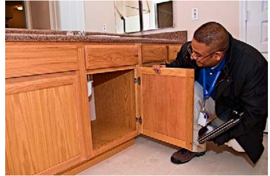
TDHCA compliance staff member Daniel Valles inspects plumbing facilities in a rental unit to ensure there are no leaks.
